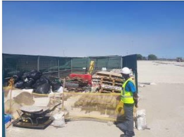
Image 16: Storage of waste within the site camp.
