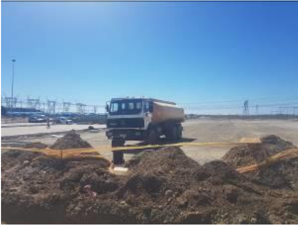
Image 13: Demarcation of excavation and construction vehicle.
