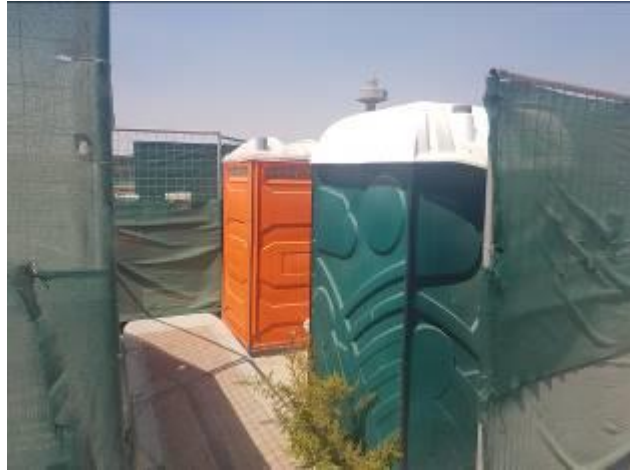
Image 25: Ablutions on site.
