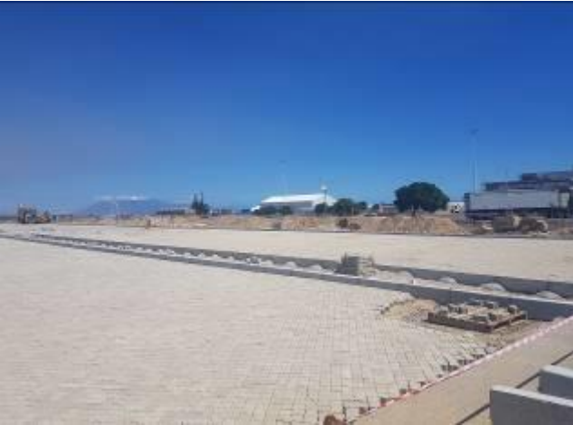
Image 19: Progress on site.
