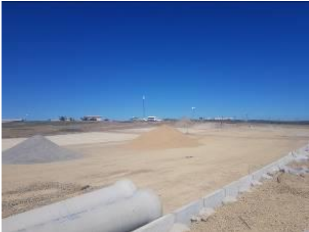
Image 12: Storage of materials on site.
