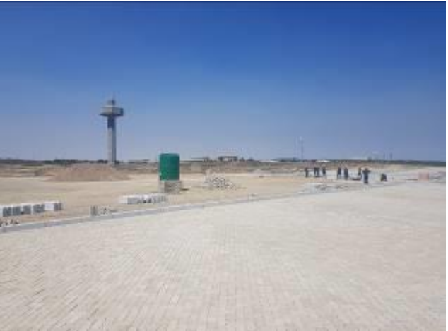
Image 22: Completed paving and cleared area.
