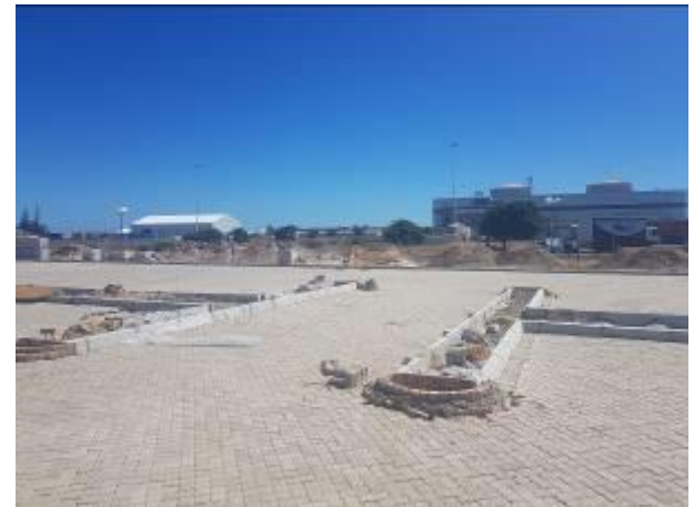
Image 6: Curb and paving laid in some areas.
