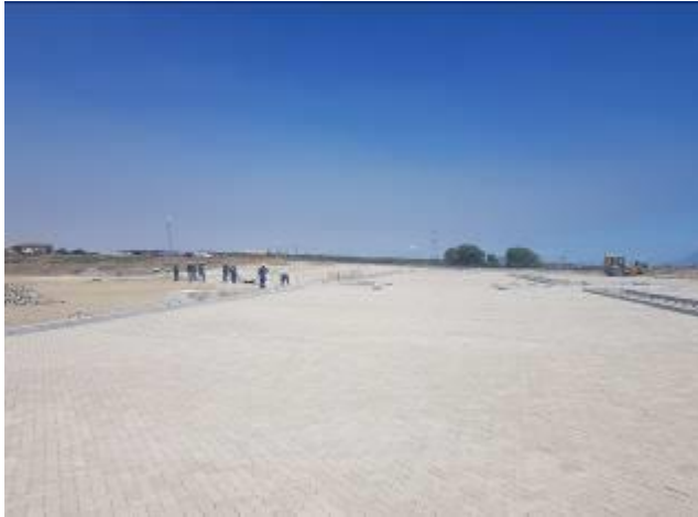
Image 20: Site seen to be in an orderly state.
