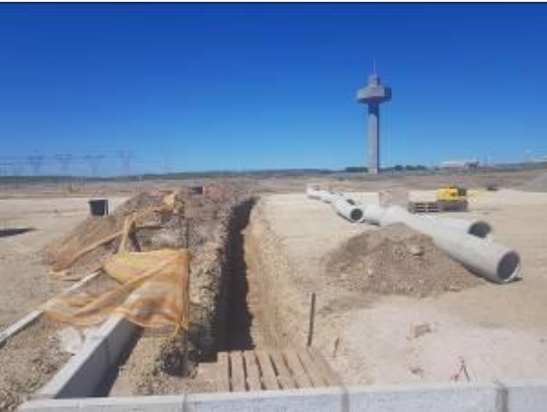
Image 10: Excavations and demarcation on site.
