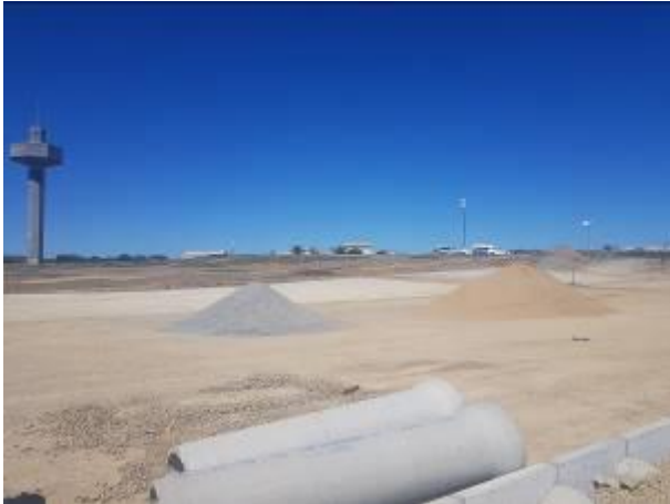
Image 9: Storage of materials on site.
