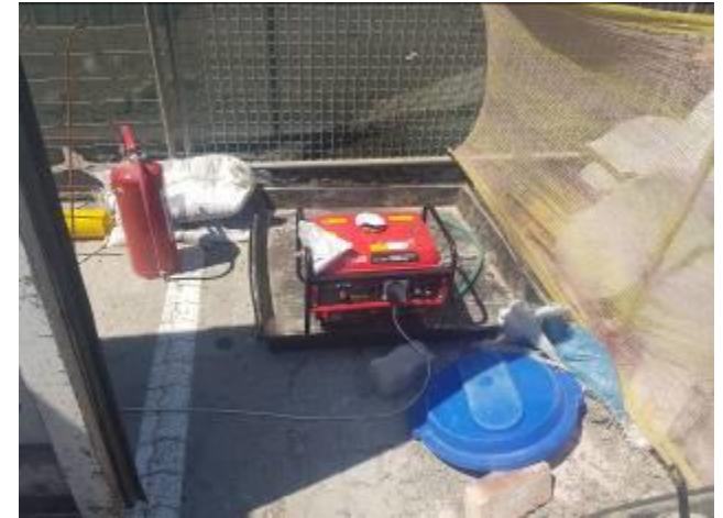
Image 17: Use of a generator and drip tray.
