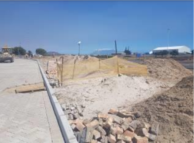
Image 21: Demarcation of excavations.
