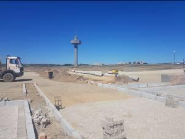
Image 7: Laying of paving on site.
