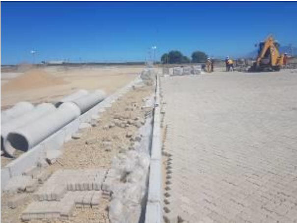
Image 11: Excess wrapping not disposed of noted on site.
